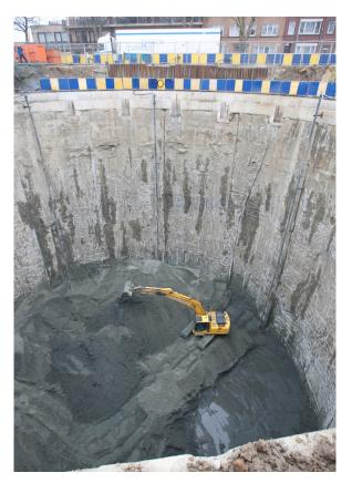
07 Excavations of a storm basin by the earthworks company De Meuter in Brussels. The Ypresian geological layer, a cohesive clay, is laid bare, and is one of the resources that BC materials uses to make building materials. (Photo: De Meuter)
